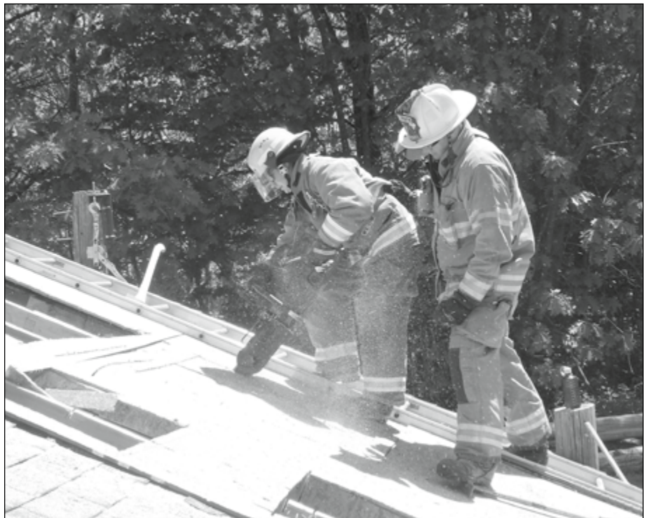
State Fire Instructor Chris Poremby - Instructing Ventilation Practices Submitted photo)
